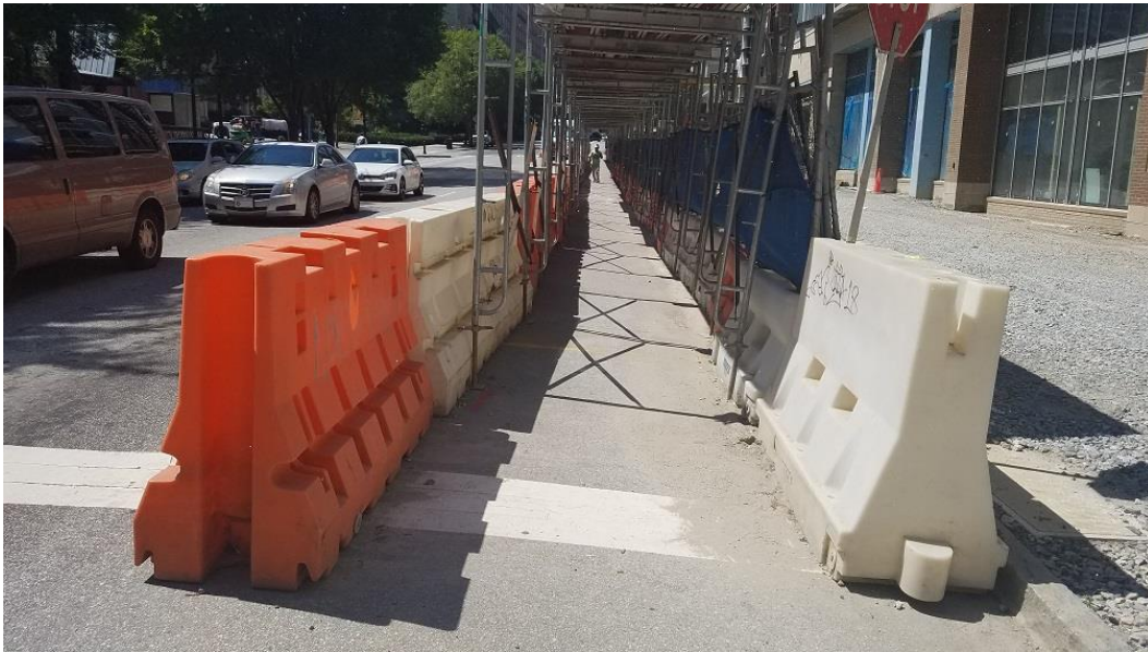
Covered Walkway on Roadway
