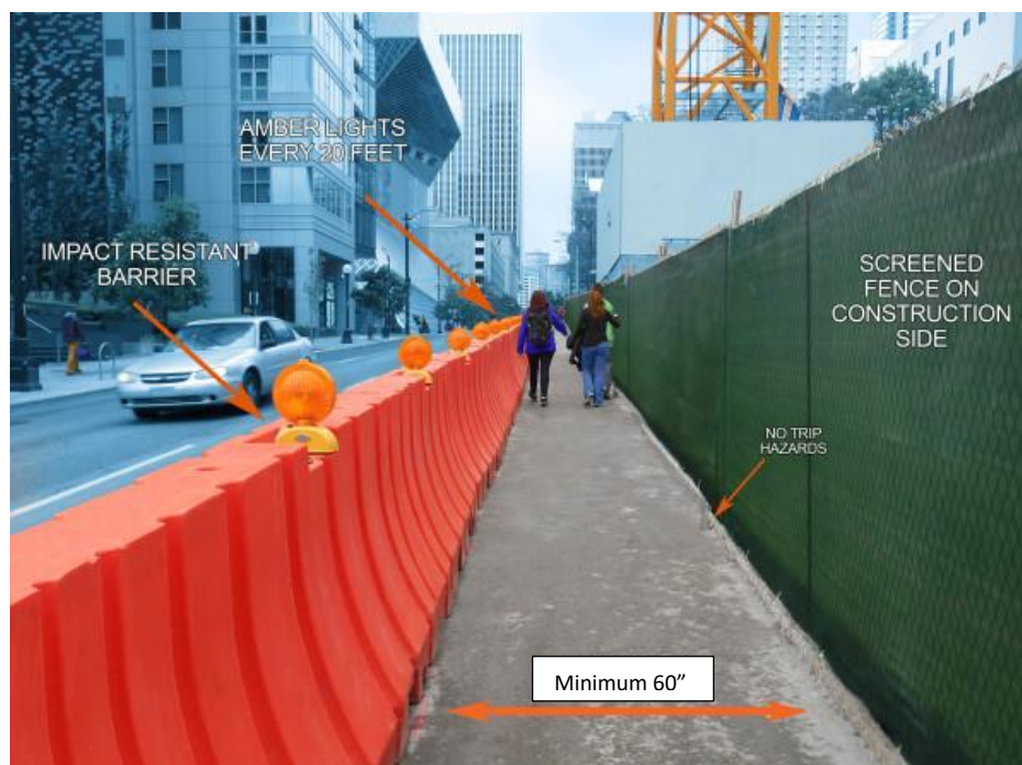
Opened Walkway on Roadway
