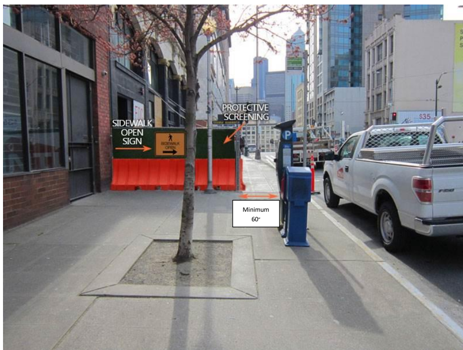
Opened Walkway on Sidewalk
