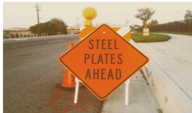
Figure 6 – Metal Plate Flashing Light
